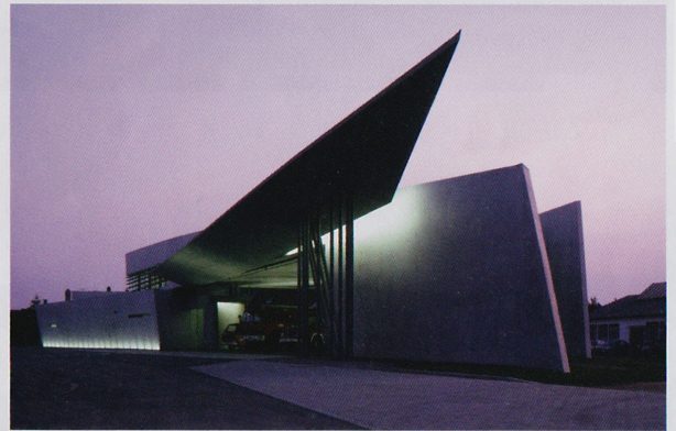
Photo: Christian Richters ©Zaha Hadid Architects
