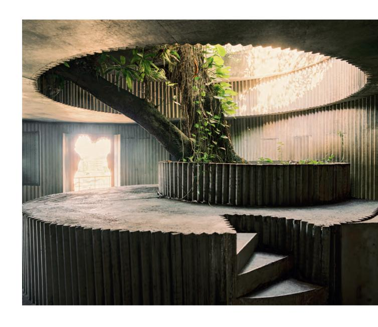
Opposite, top left: a clash of concrete, trees and ruin – the entrance to Coati via wrought-iron doors. Top right: with engineer João Filgueiras Lima, Bo Bardi developed a modular system of corrugated concrete to stabilise the restaurant's old and new structures. This page: a mango tree dramatically pierces the building's dining area
